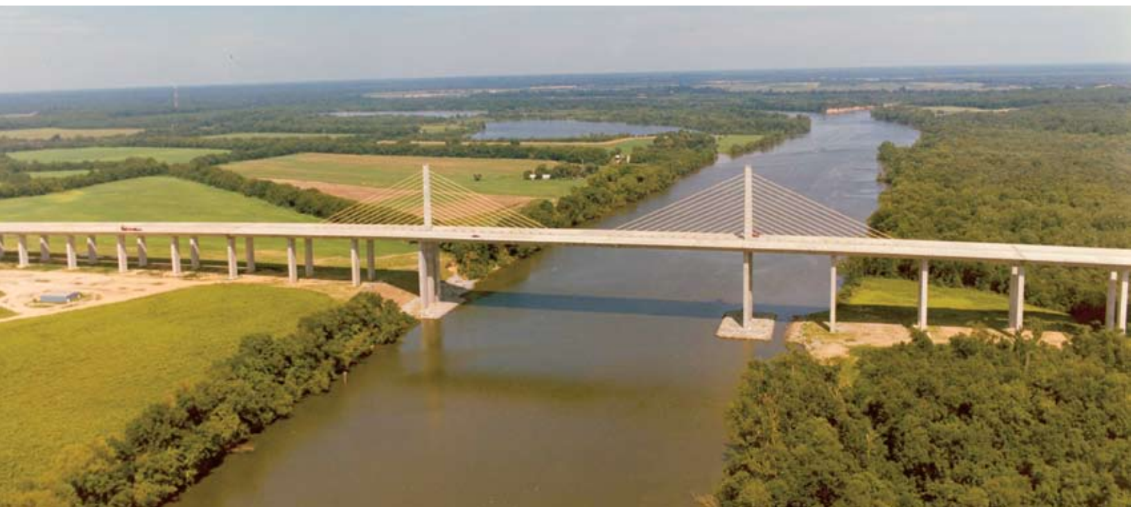
The Varina-Enon Bridge on I-295 near Richmond
